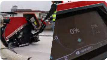
Abrasive flow controlled by Digisteer
